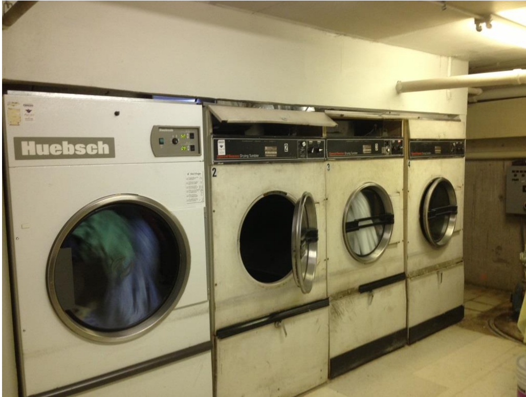
Figure 4: Healthcare Facility Dryers (2 on left were monitored and retrofitted)
