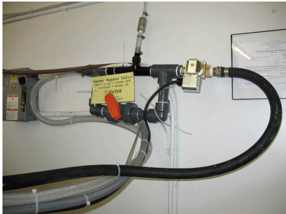
Figure D-4 Detail of Ozone Supply Line (top) and Venturi Connection with Cold Water Supply
