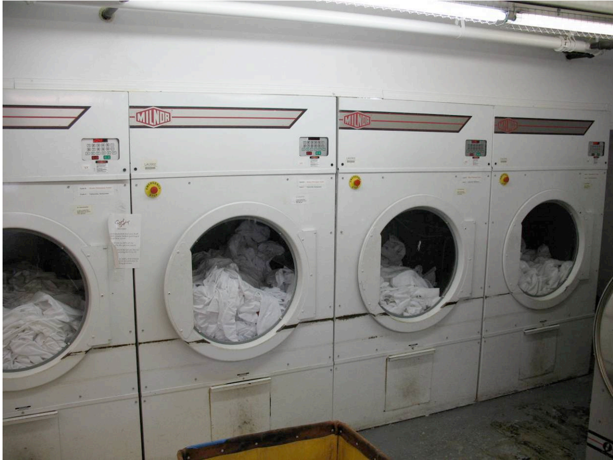
Figure D-2 Four Pellerin Milnor Model MLG130HS 120 lb Gas Dryers
