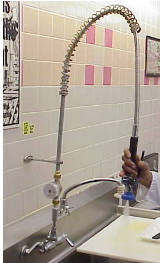
Figure 3: Metering setup for determining hours of use
