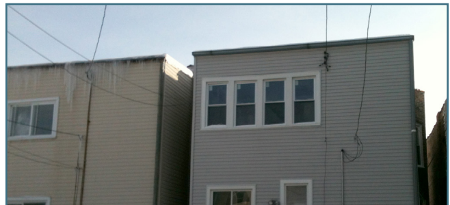
Liz Vogel's home (above right) is now free of the ice dams seen on a neighboring building (above left).
