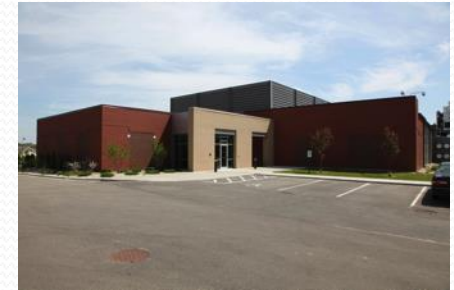
Utility "Back Office"
