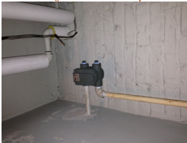
Figure 7-5: ERP-03 Steam Trap
