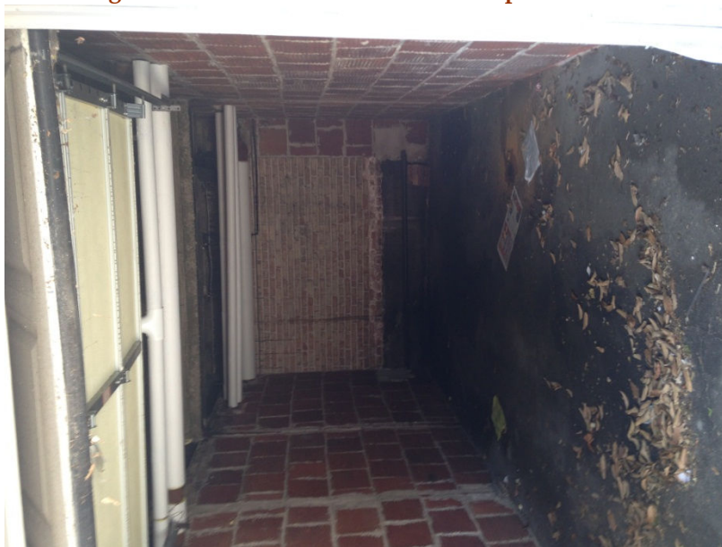
Figure 7-7: ERP-05 Steam and DHW Pipe Insulation
