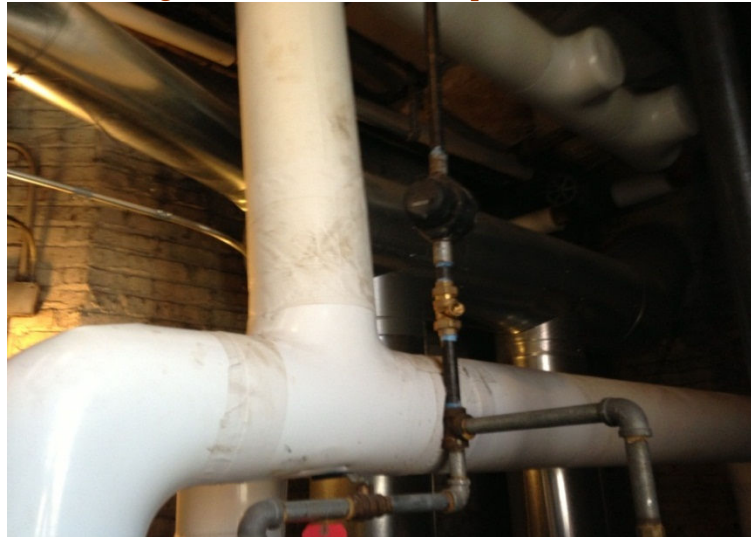
Figure 7-4: ERP-03 Steam Pipe Insulation
