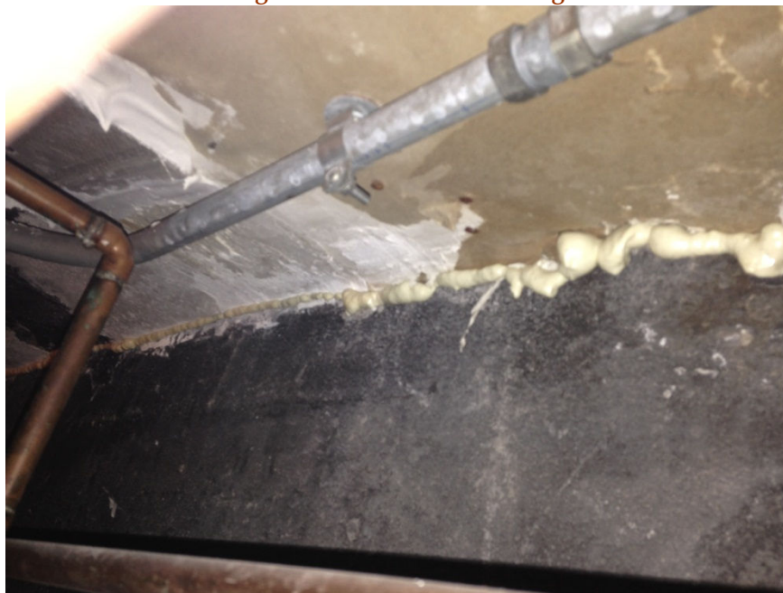
Figure 7-3: ERP-02 Air Sealing
