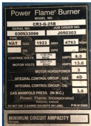
Figure 7-6: ERP-05 Power Flame Burner Nameplate
