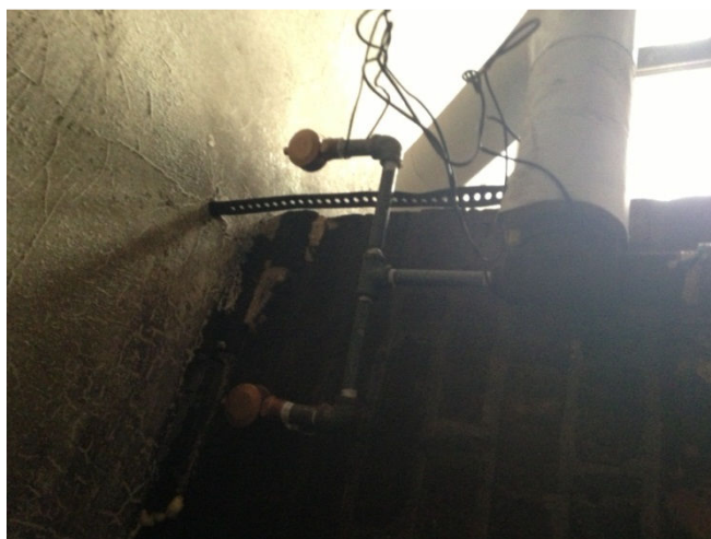
Figure 7-1: ERP-01 Steam Vents
