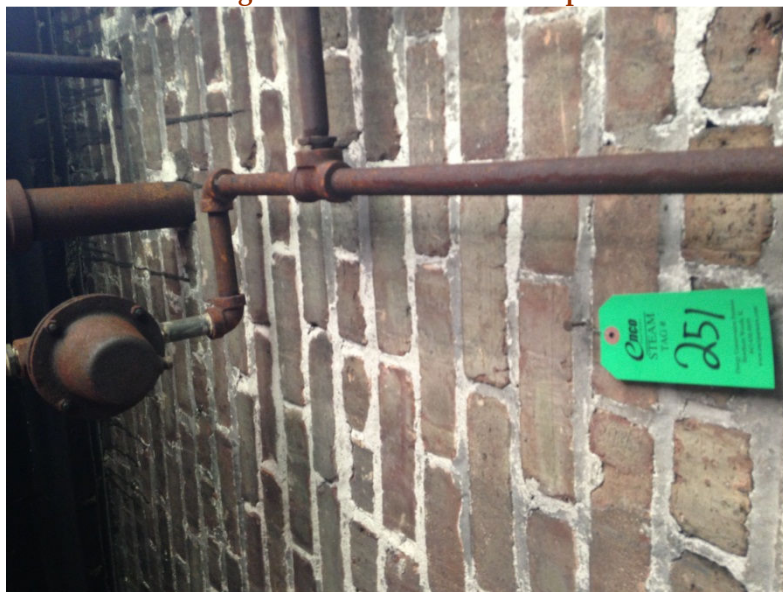
Figure 7-8: ERP-05 Steam Trap
