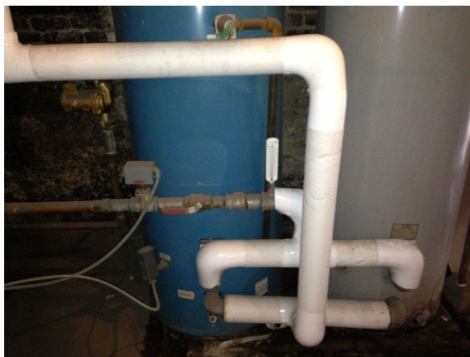
Figure 7-2: ERP-01 DHW Insulation
