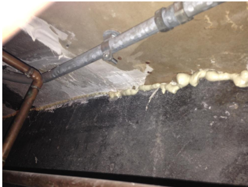
Figure 3: ERP-02 Air Sealing
