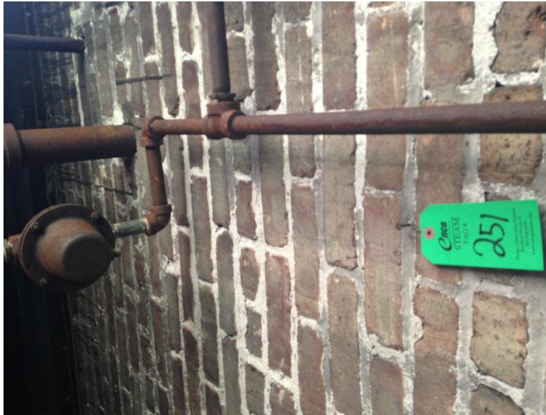
Figure 8: ERP-05 Steam Trap
