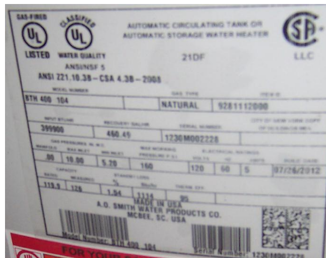
Figure 10: ERP-12 Water Heater Nameplate
