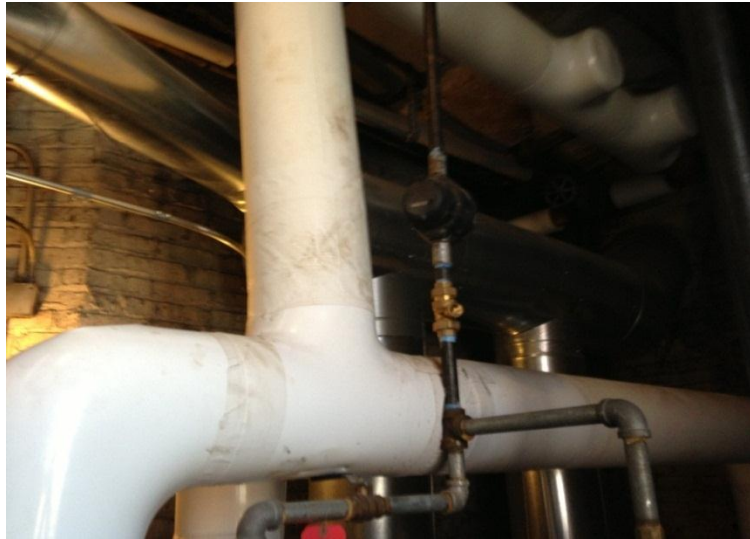
Figure 4: ERP-03 Steam Pipe Insulation
