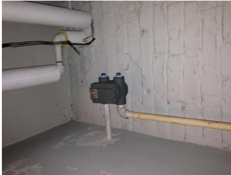
Figure 5: ERP-03 Steam Trap
