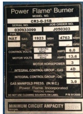
Figure 6: ERP-05 Power Flame Burner Nameplate
