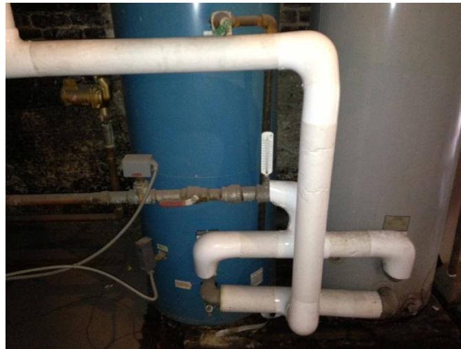
Figure 2: ERP-01 DHW Insulation
