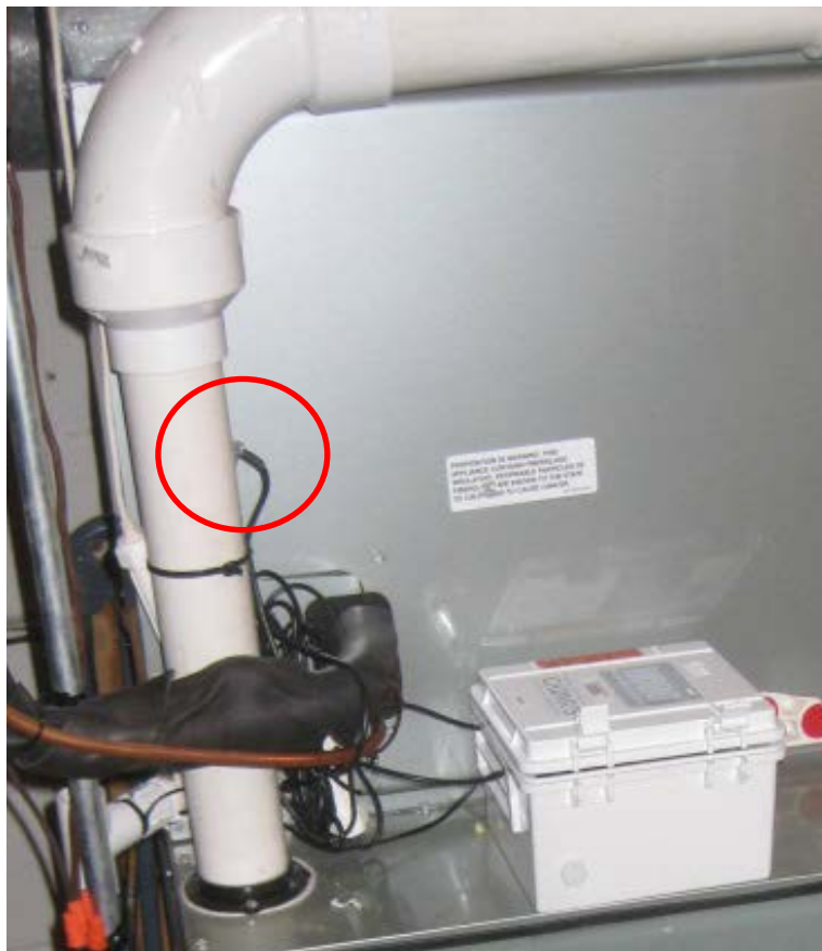
Figure 31. Temperature Sensor in Flue Gas Pipe
