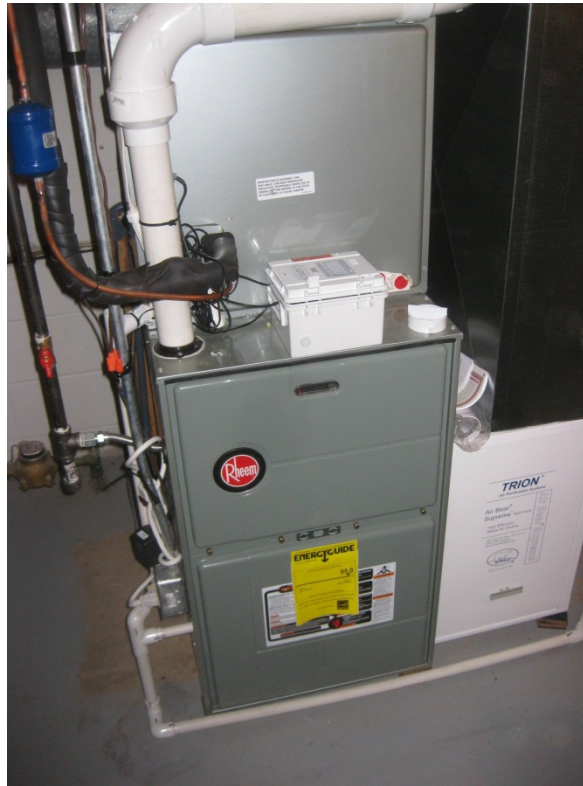
Figure 28. Cellular Logger for Furnace and AC Meter Installation
